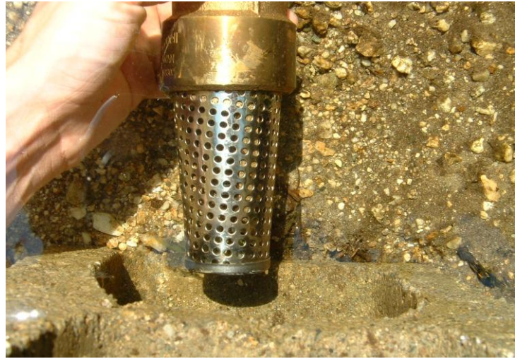
Figure 2. Diversion screened to keep debris out, but not fish.
