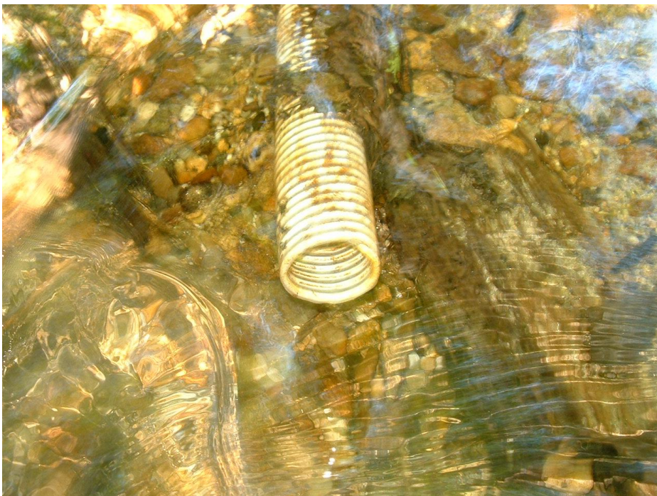
Figure 1. Unscreened diversion on East Fork Smalle Creek (Site No. 1520106)
